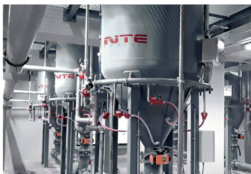
DENSE PHASE CONVEYING WITH TRANSPORTERS M201
