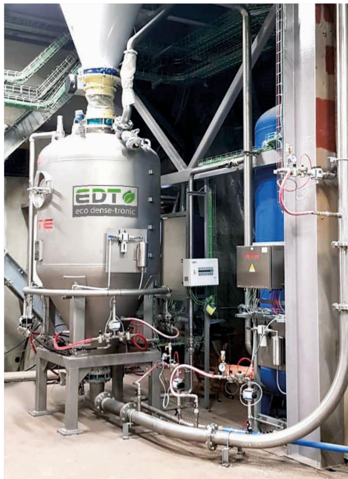
TYPICAL ECO DENSE-TRONIC® INSTALLATION
